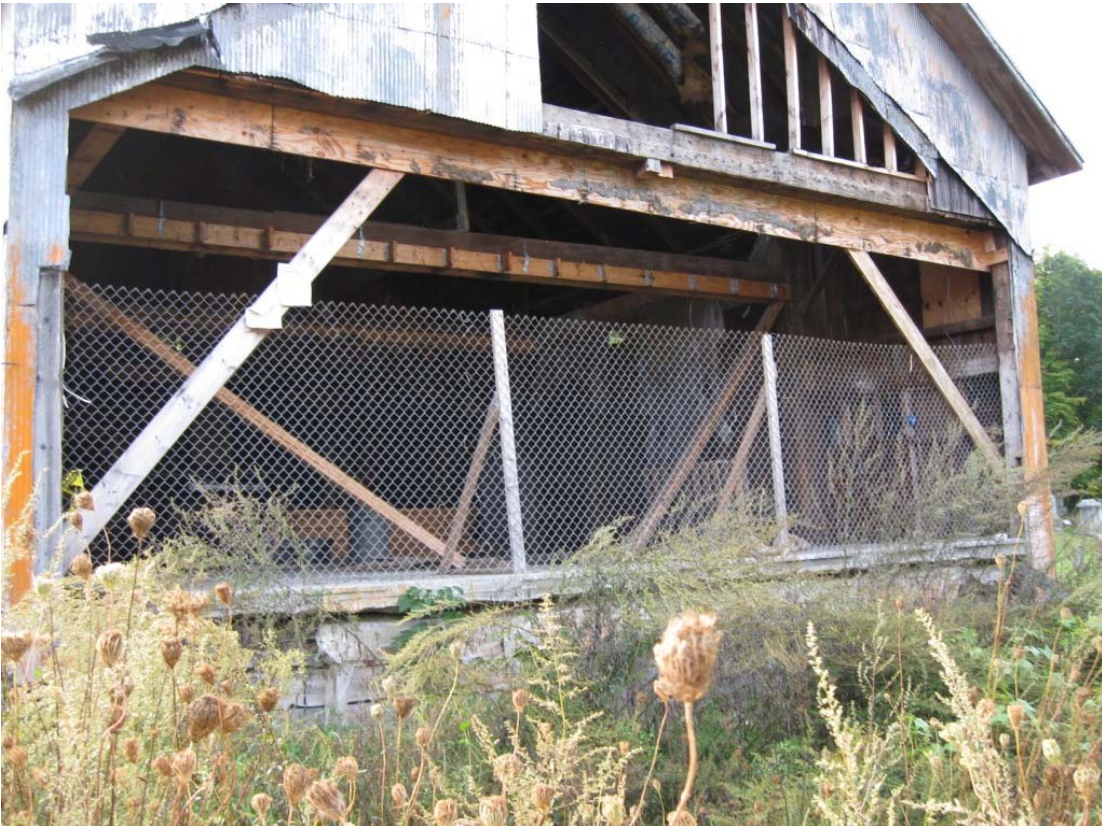
Plate 2: Former cooler storage building
