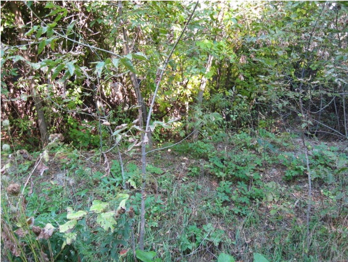
Plate 5: Berm covering wastewater conveyance pipe
