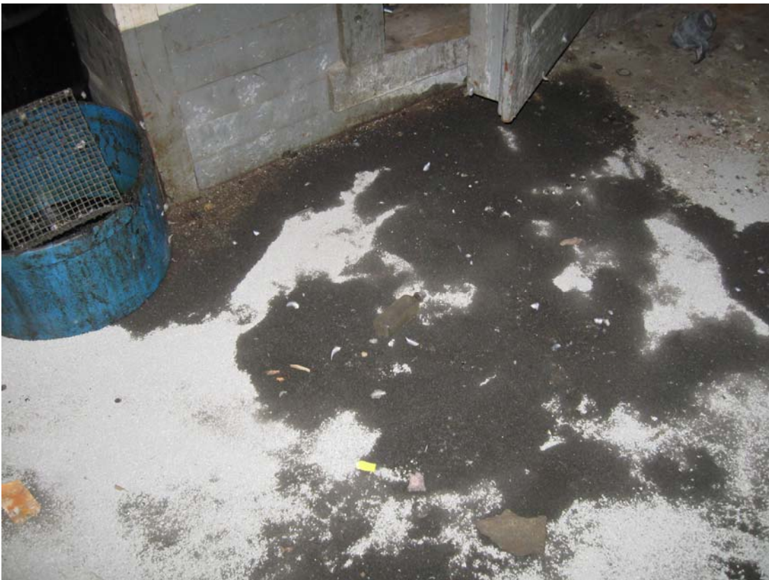
Plate 14. Oil spilled on Level 1 by vandals.
