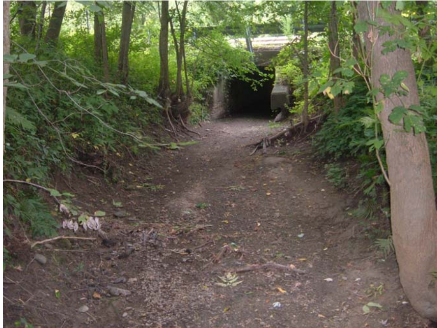
Figure 7. Dry channel below Rt. 2 box culvert in reach R9.S2.01
