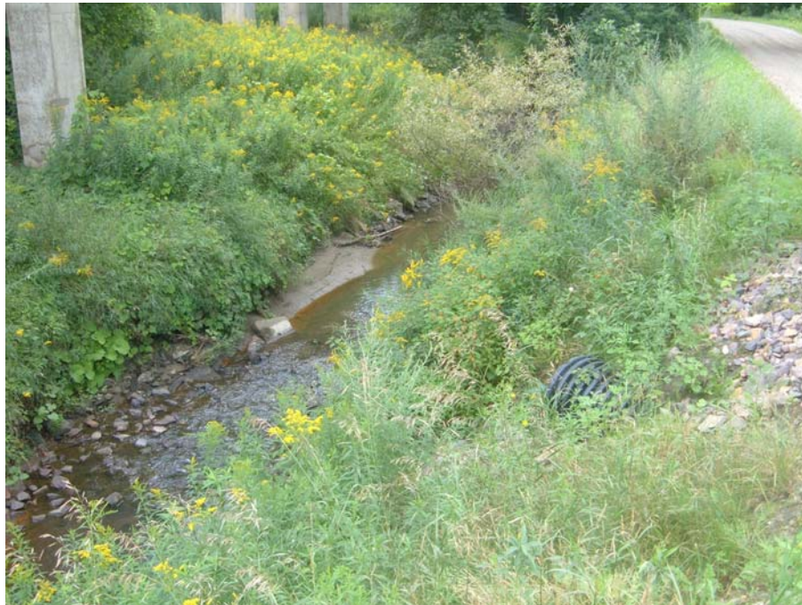
Figure 3. Stormwater outfall and lack of woody vegetative buffer in R8.S1.01
