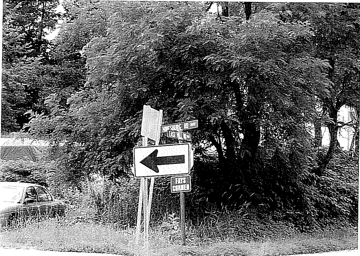
Figure 14. SIGN ASSEMBLY NEXT TO EAST HILL RD PROVIDES TOO MUCH INFORMATION
