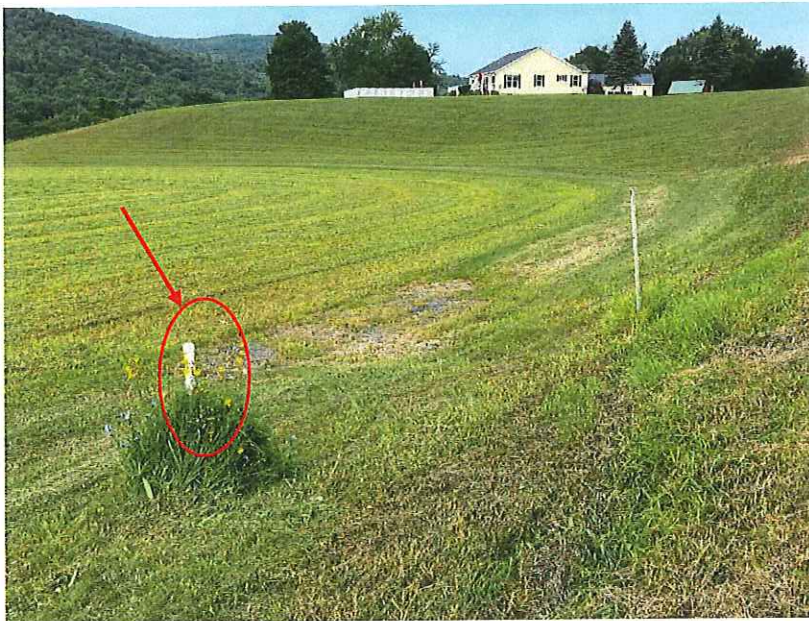
Figure 1 - White post and culvert marker post shown
