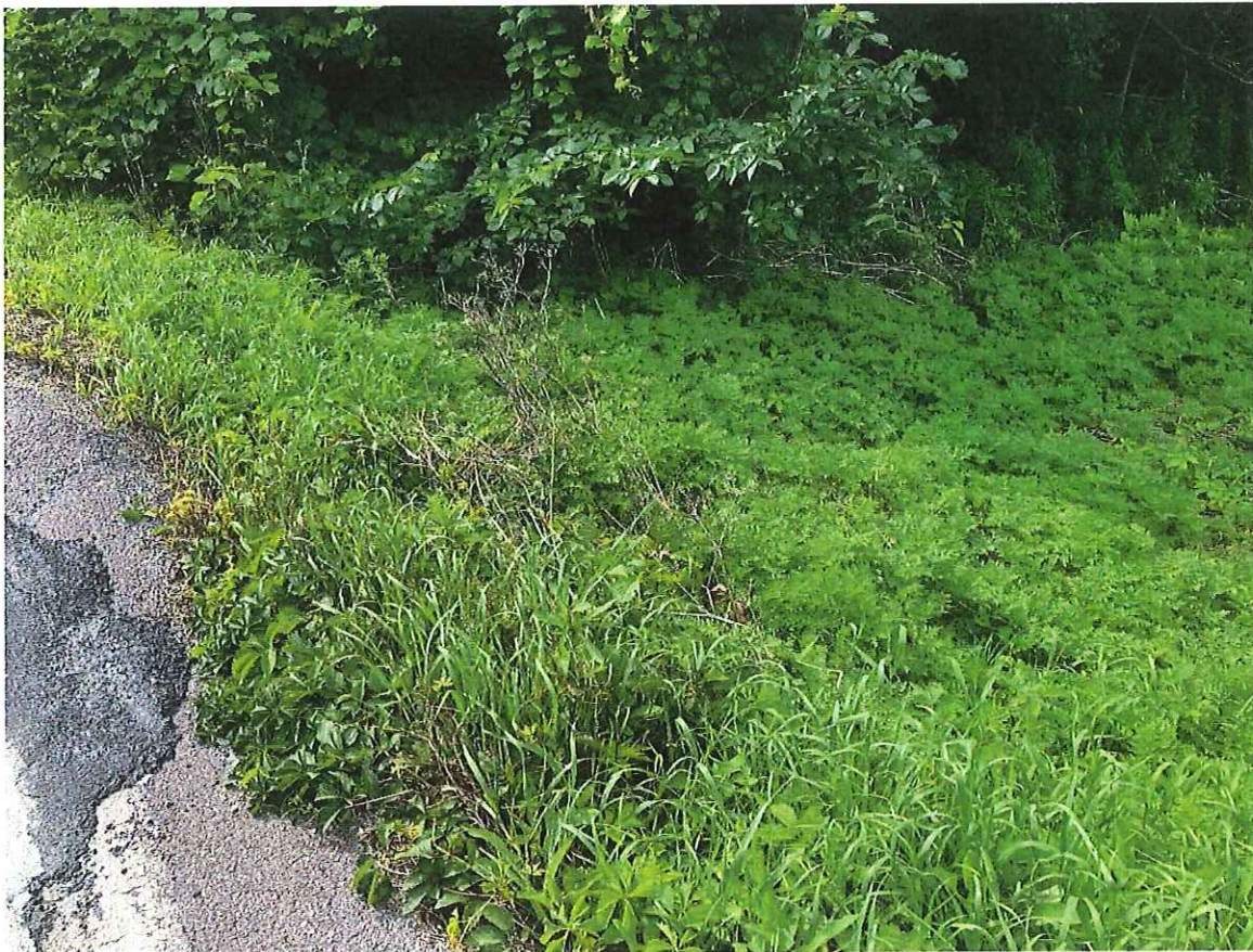
Figure 1 - Slope to fix on EB side road ~10ft from outlet
