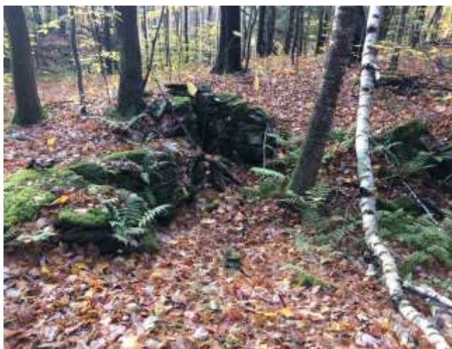
One of the old foundations on the site. (Photo by Lou Borie)
