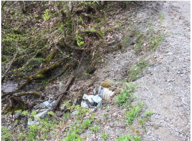
Photo 2: Existing undersized culvert and downstream gully erosion.
