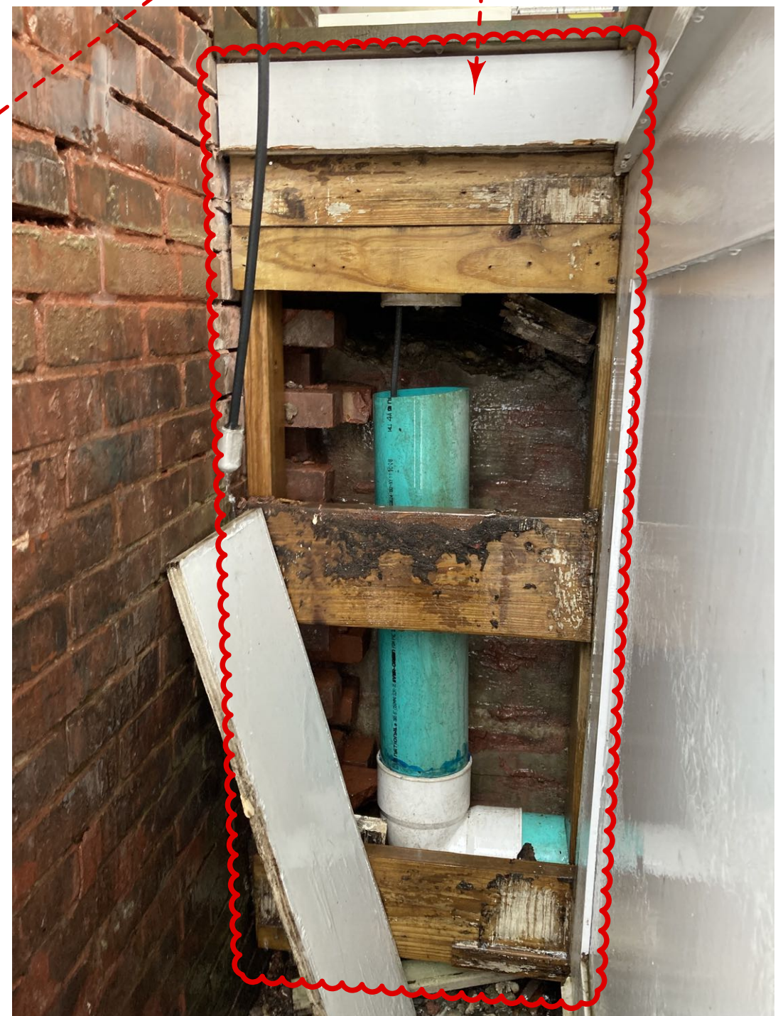
PORCH SKIRT PANEL (CURRENT CONDITION)
