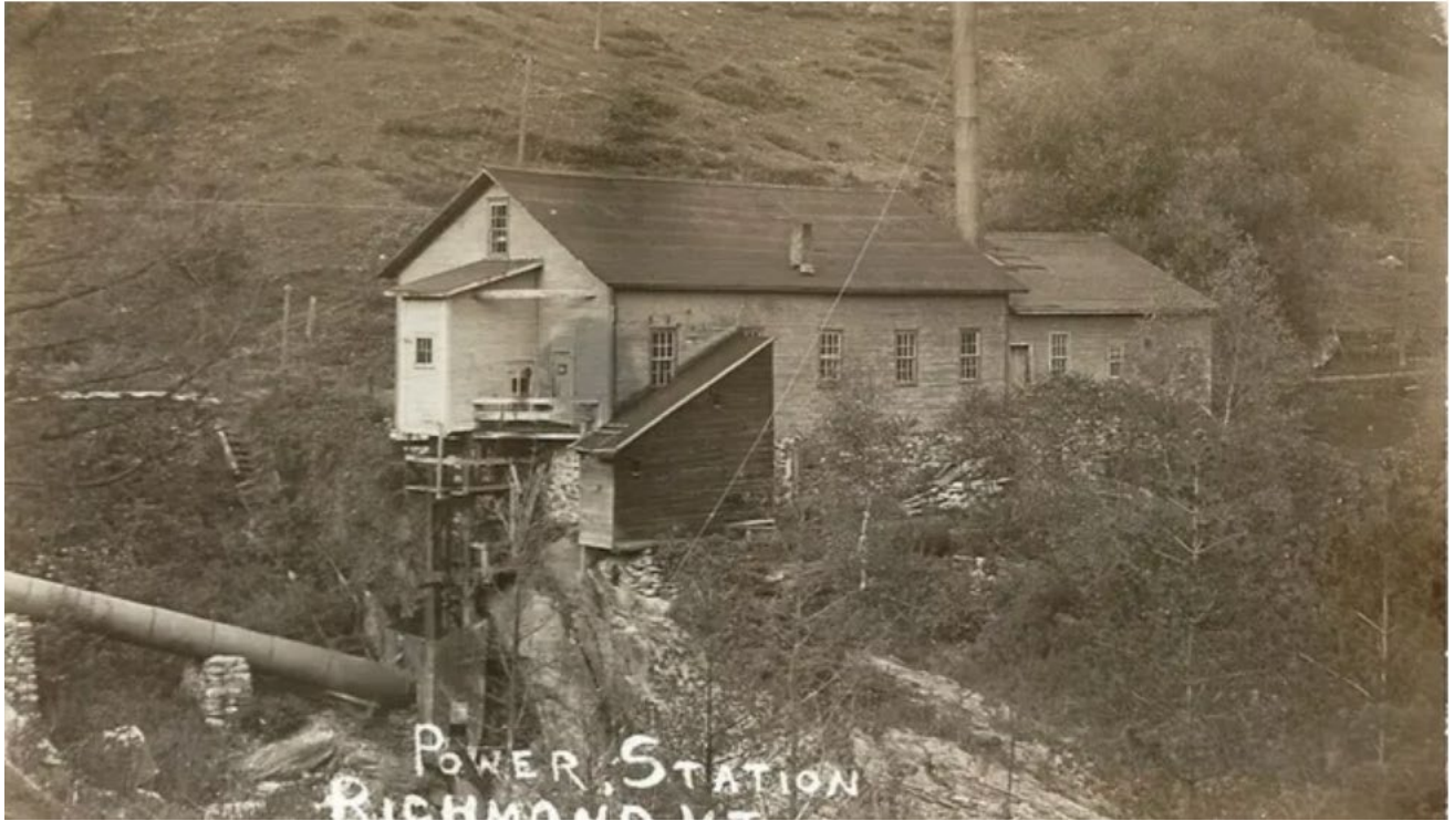
Figure 8. Photograph of the Richmond Light and Power hydroelectric plant at Huntington Gorge ca. 1905 (from Turner and Low 2015 where author's note that the image is courtesy of Ed Neuert). Note project area lies to the left of the building.
