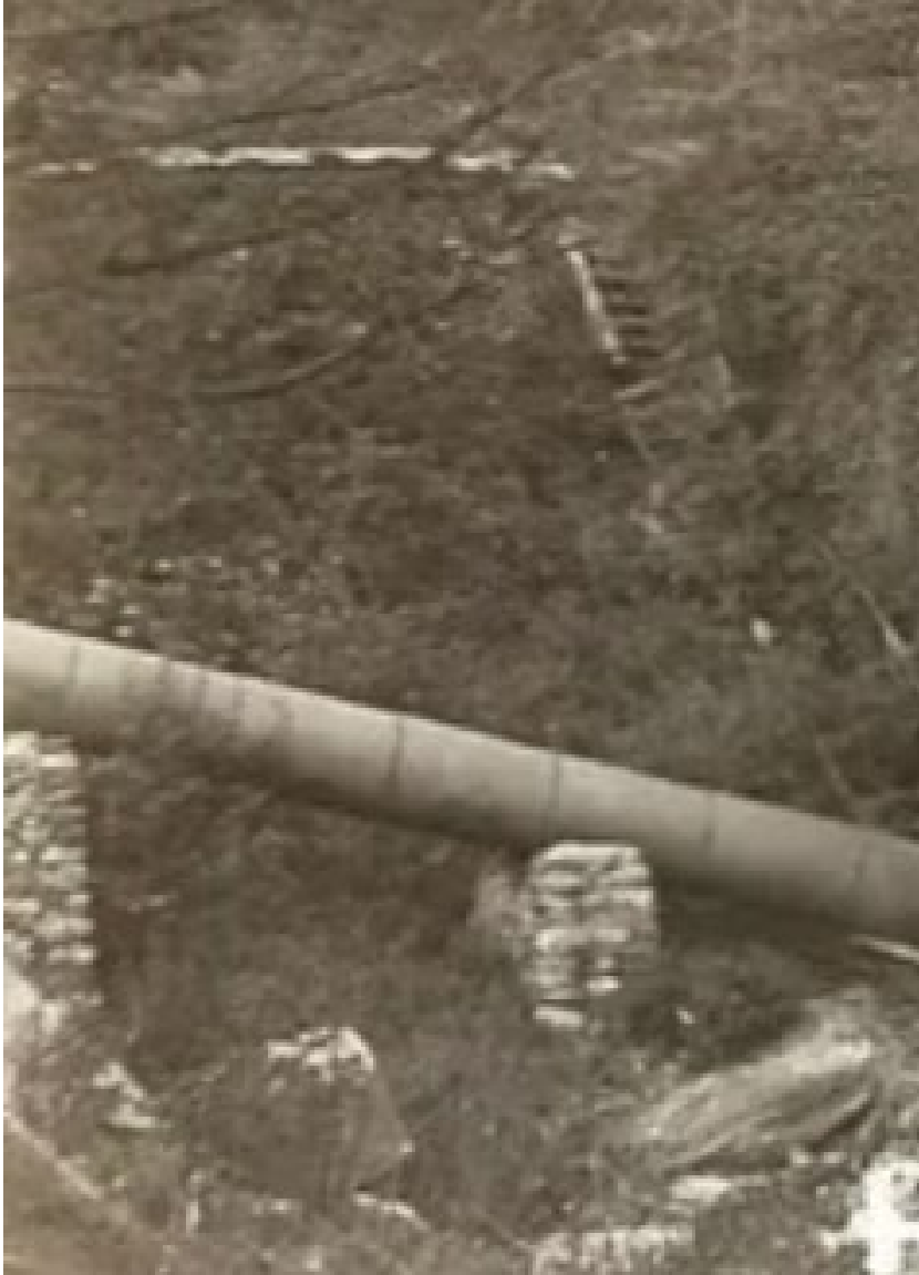
Figure 10. Close-up of historic photograph of the Richmond Light and Power hydroelectric plant at Huntington Gorge shown in Figure 8 (from Turner and Low 2015 where author's note that the image is courtesy of Ed Neuert). Note penstock abutment at left which is visible at the base of the current Dugway Road slump. Evidence of the smaller abutment at center is not immediately apparent.
