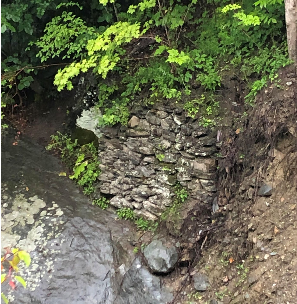
Figure 9. Stone masonry feature at the base of the Dugway Road slump, likely the remains of a penstock support dating to the use of the adjacent property by the early twentieth century Richmond Light and Power hydroelectric plant.
