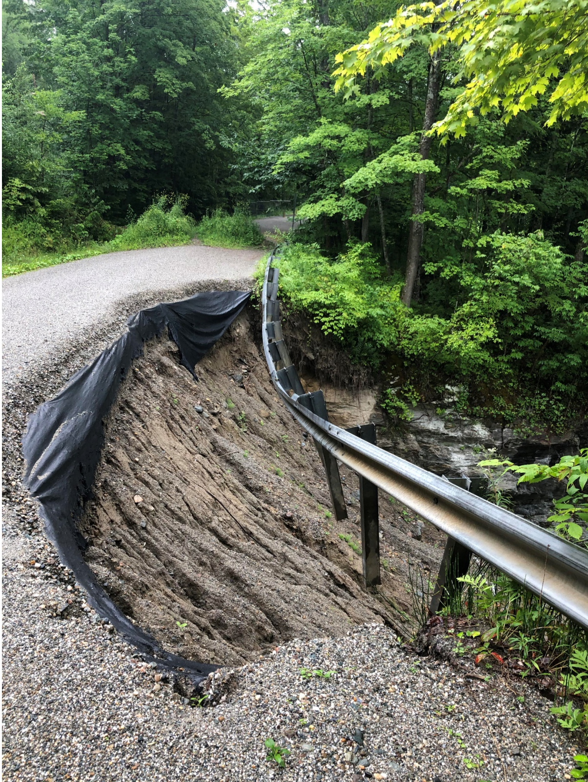
Figure 2. Photograph of the Dugway Road slope failure and project area, facing east (8/4/20).
