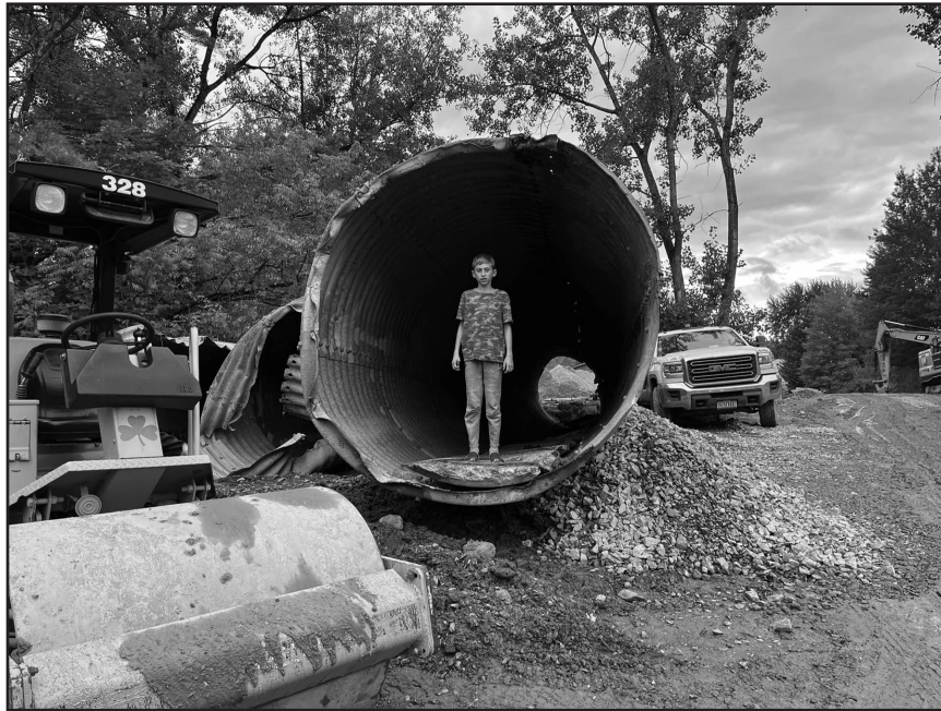
Standing in the I-89 culvert.
