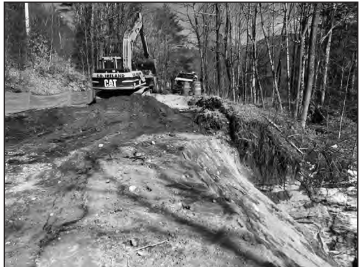
Work on the reconstruction of Dugway Road.
