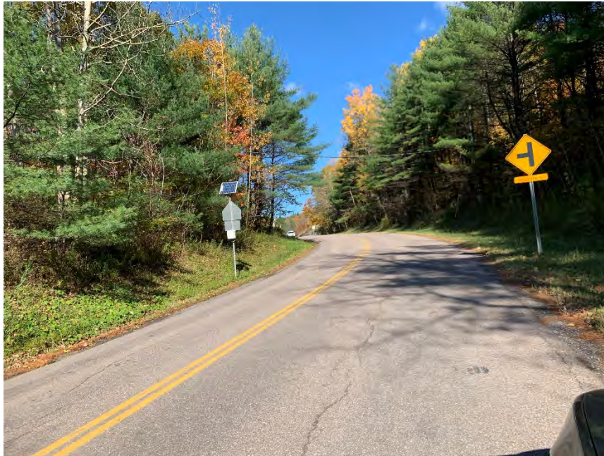
Photo 1. Project Area 1 looking north on Jericho Road
