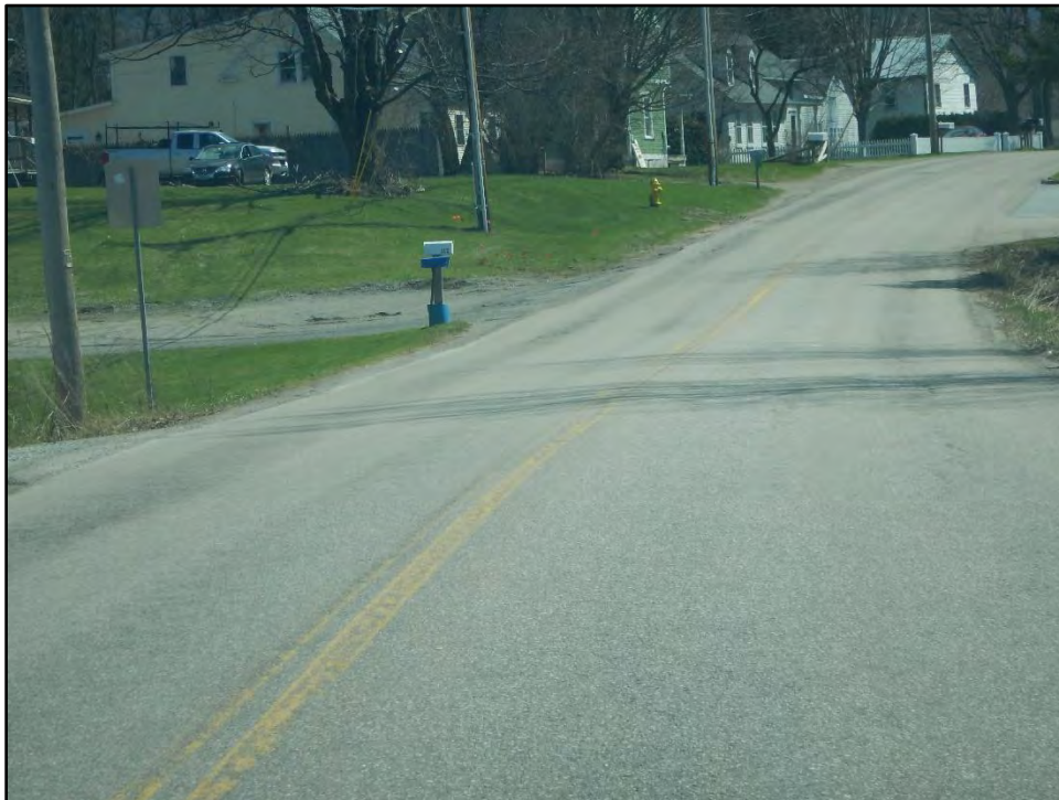
Photo 1. Photo shows the historic houses located on the eastern end of the Huntington Road project alignment. View is to the east.
