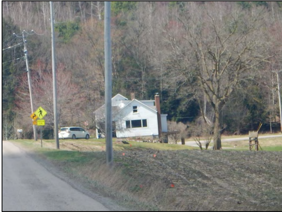
Photo 4. Photo shows the farmstead located at the bend in the road near the western end of the Huntington Road alignment. View is to the west.
