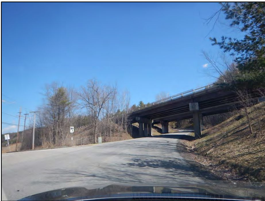
Photo 9. Photo shows the southern end of the Jericho Road alignment at the intersection with School Street. View is to the north toward the I-89 overpass.
