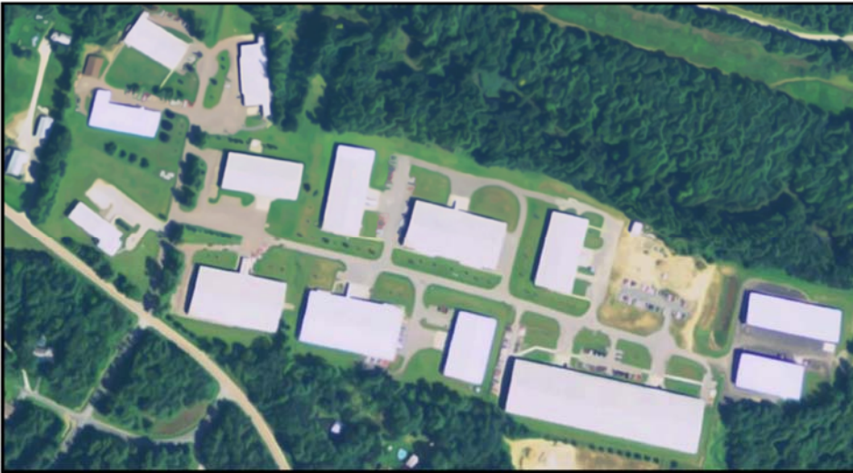
FIGURE 8: Efficient Use – Industrial Example
