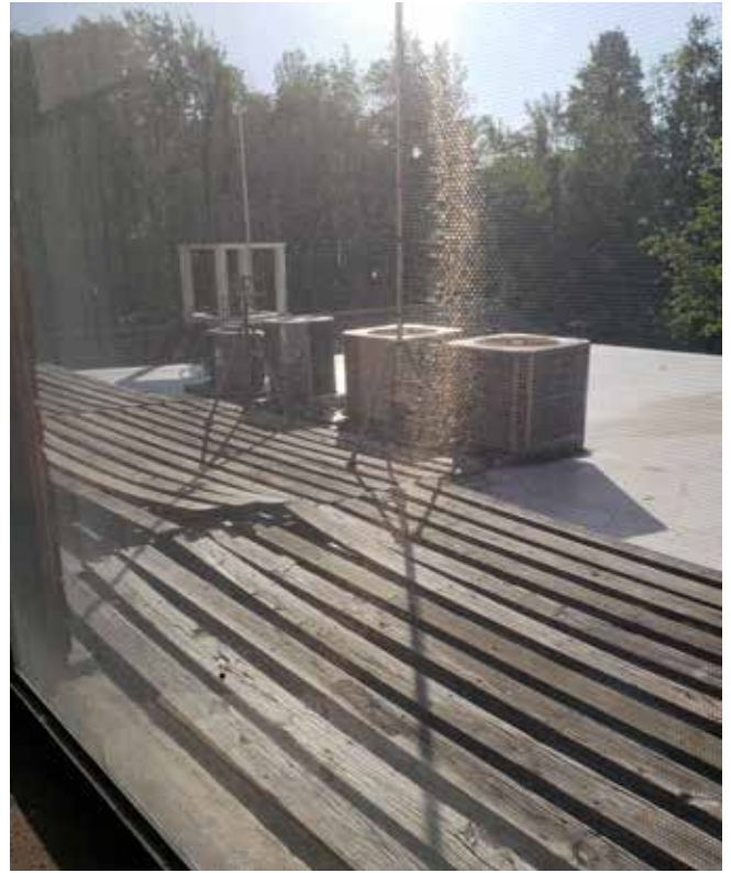
Photo of Post Office roof
