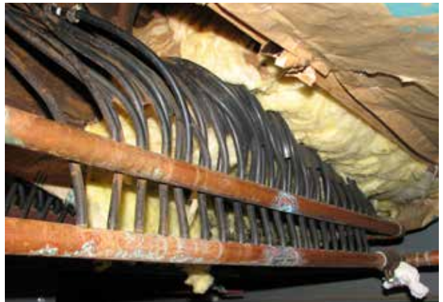
First floor radiant heat piping
