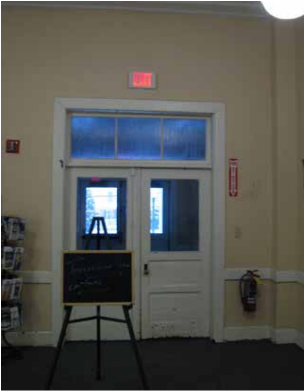
First floor lobby Bridge Street entrance
