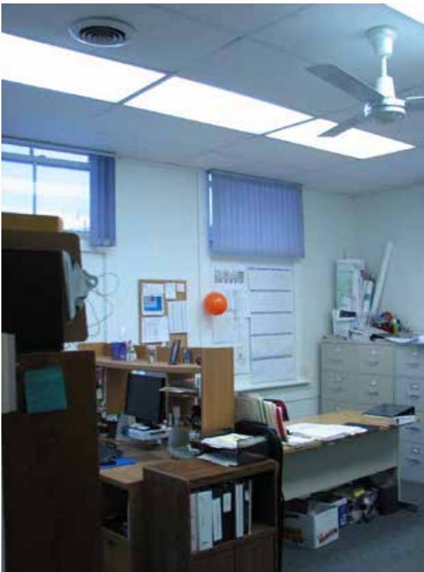
Zoning Office - Infill panels over windows
