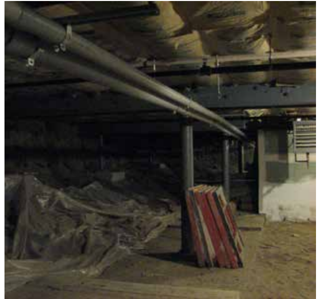
Dirt floor at basement level
