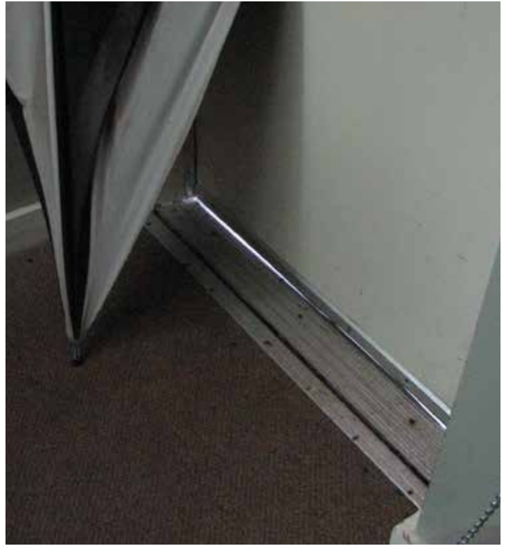
Daylight at stair tower door
