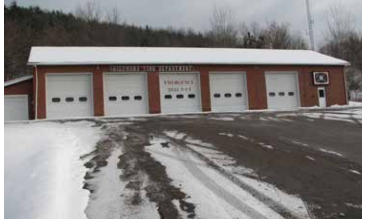
Steep apron approach from Route 2
