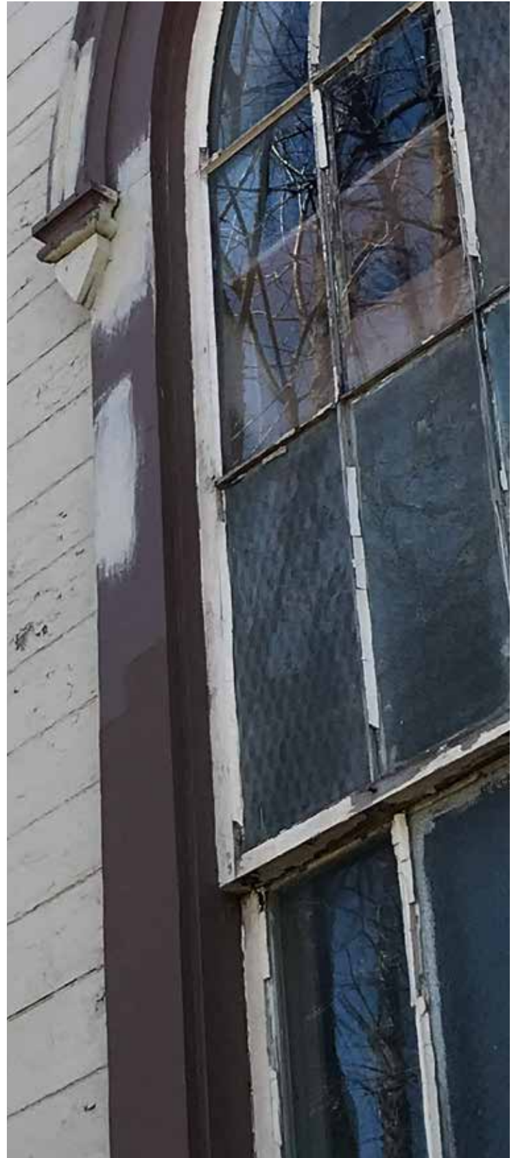
Community Room window exterior
