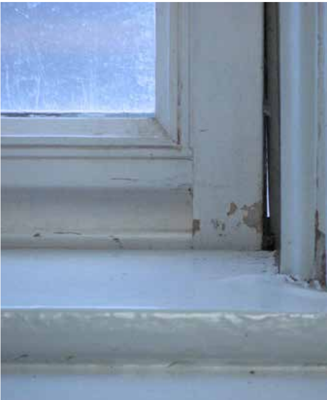
Daylight at window frame
