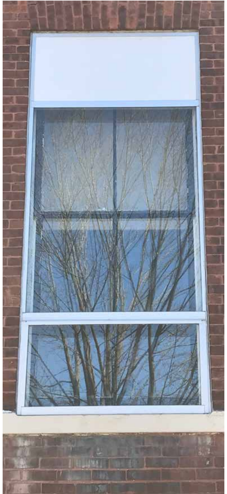
Window exterior elevation photo
