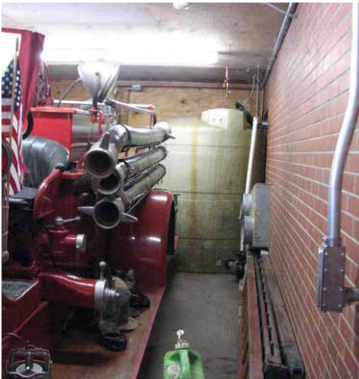
Existing, undersized truck fill tank
