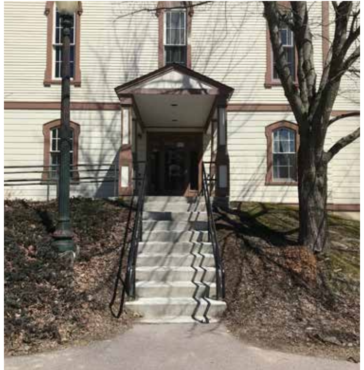
Stairs at main entrance
