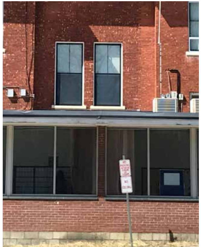
Post Office storefront and soffit
