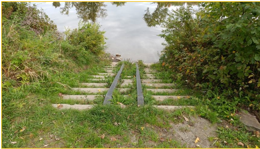
Figure 6. Another stair design example with boat ramp several years after installation.
