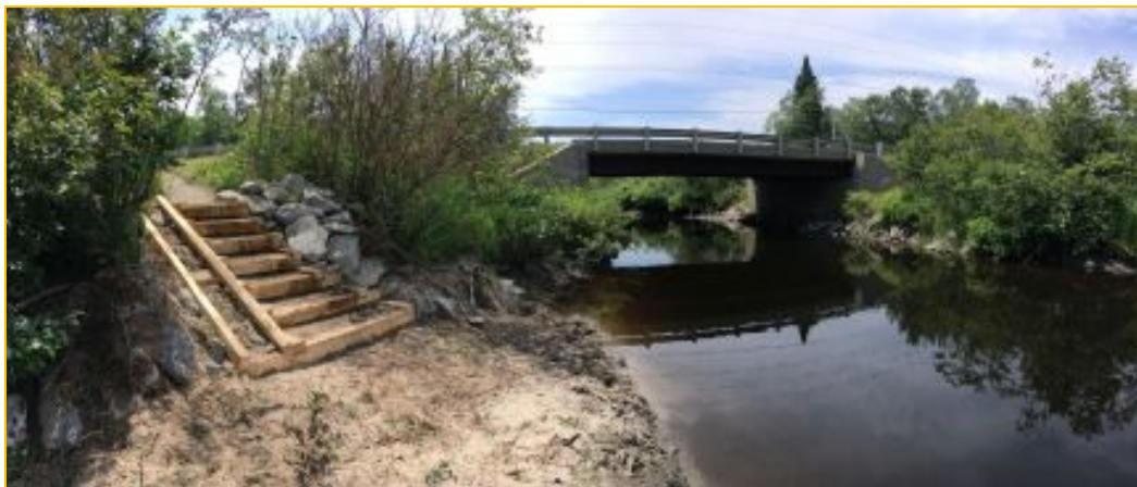
Figure 5. Example of stairs with boat ramp shortly after being installed
