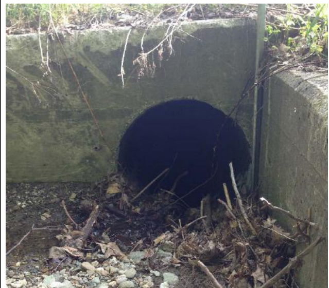
Photo 2. Culvert inlet intercepting intermittent stream flow and upland runoff from the F2 drainage and conveying it beneath I-89.
