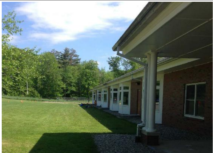
Photo 1. Proposed rooftop disconnection area, also showing existing gutter and drain system for roof fumoff.
