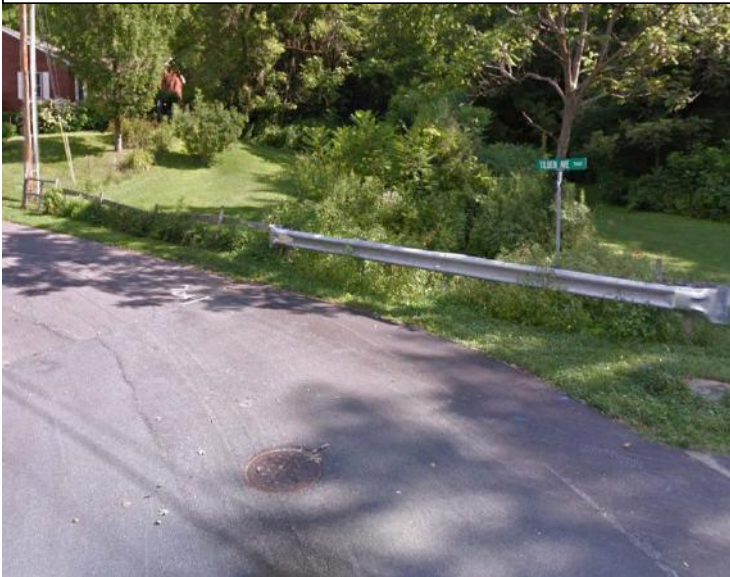
Photo 1. Corner of Millet Street and Tilden Avenue where stormwater enters the closed drainage system
