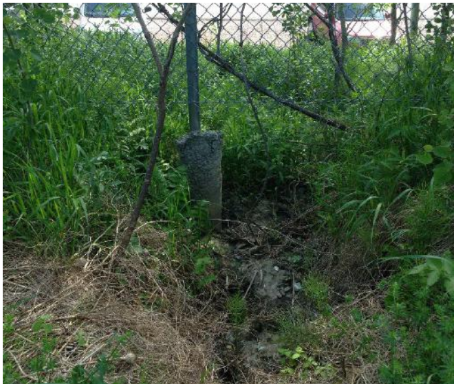
Photo 1. Gully erosion downslope of culvert outlet, leaving I-89 ROW and entering USD 17 property. Note exposed concrete fence footer and chloride-damaged vegetation.
