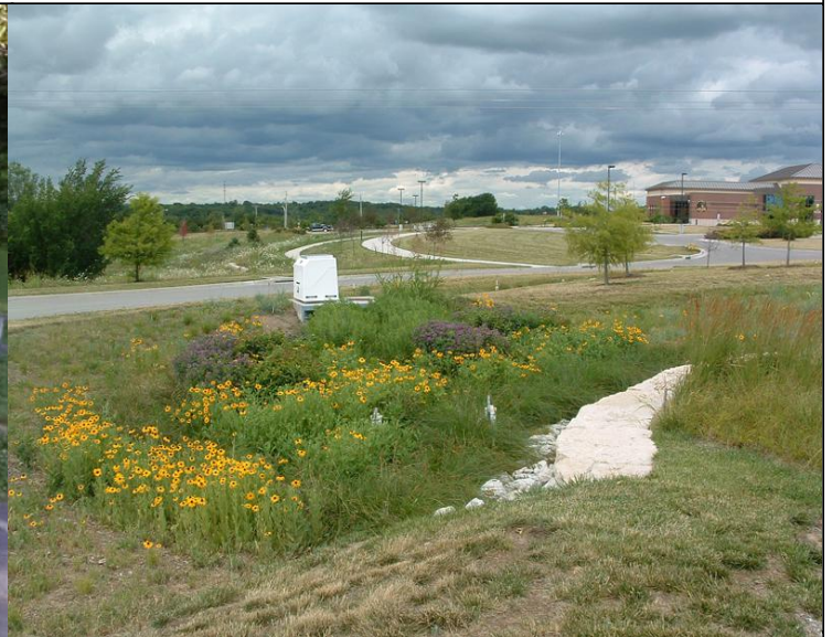
Photo 2. Typical bioretention basin
