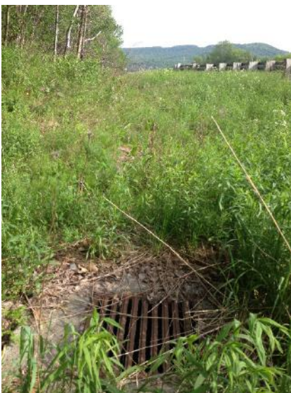
Photo 1. Potential BMP area, looking south.
