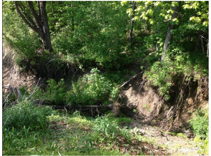
Photo 2. Same gully wall as Photo 1, showing recent erosion and a large tree toppled into the gully with leaves still green.
