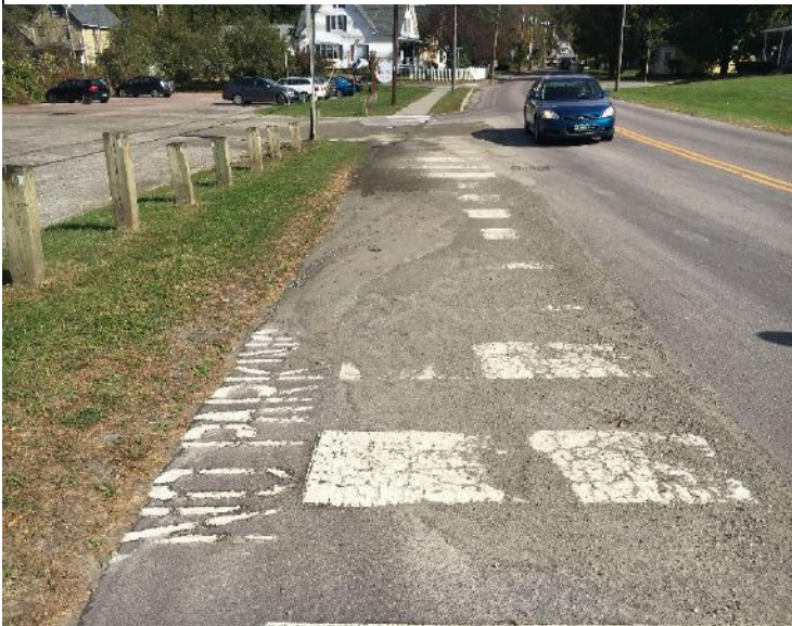
Photo 1. Entrance to the recreational fields parking lot
