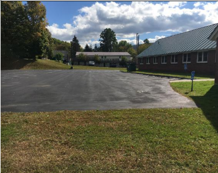
Photo 1. Parking lot and roof currently draining to green space
