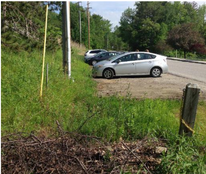
Photo 1. Existing gravel parking area; drainage swale is at left.
