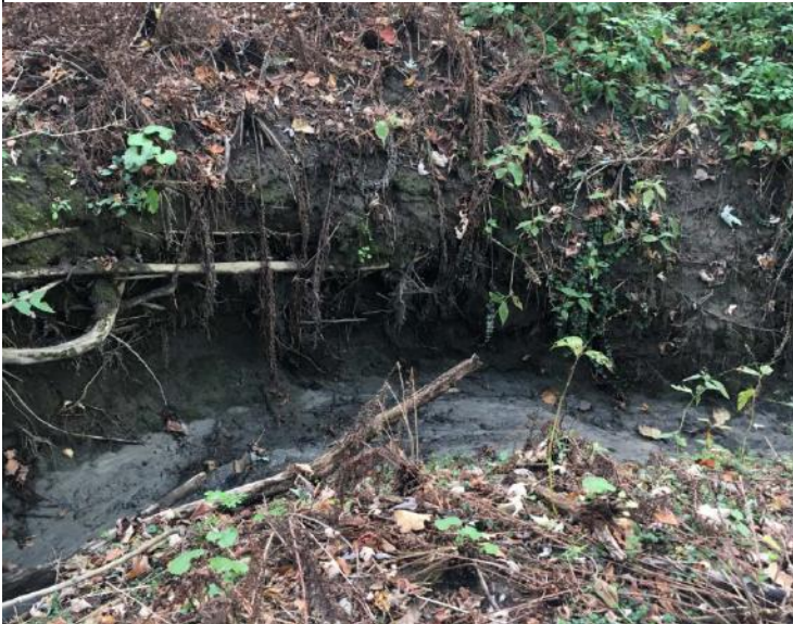
Photo 1. Eroding drainage ditch
