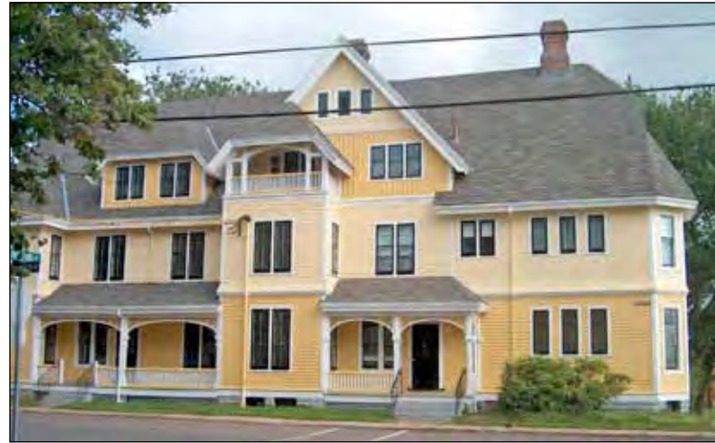
Multi-family housing can be designed to look like large single-family homes and existing large homes can be converted to multi-unit structures to increase housing opportunities in a village setting
